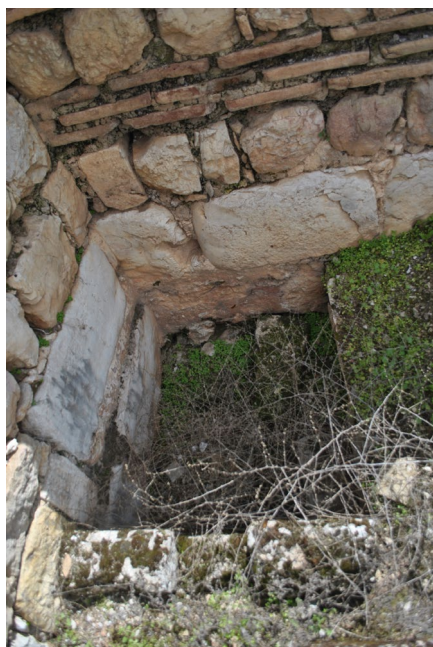
Figure 12. ‘Anjar: dār al-imāra . Remains of a tank (Photo by the author, 2017)
