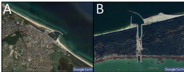
Figure 1 - A: Port of Władysławowo, B: Port of Przekop Mierzei, Poland. Examples of medium-sized semi-closed ports in the South Baltic Sea.
